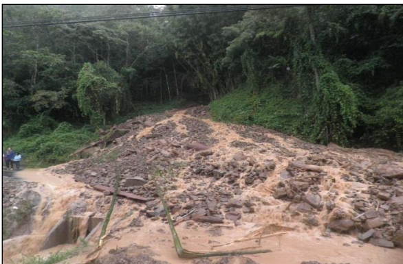
Photo 1: Debris flow at Jalan Tamparuli-Ranau KM 83.90 on 6 th May 2012
