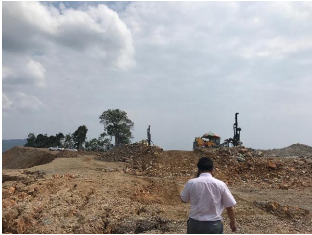
Figure 5: Drilling operation for blasting work at the top of hill.
