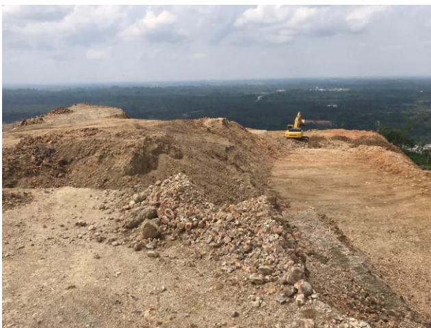
Figure 4: Top soil excavation and slope trimming in progress.
