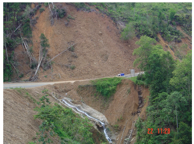
Figure 11: Wedge failure (blocks and fragments) (B3 – a) at RS 3 indicates the form of discontinuities provides intersecting sheets to form yield stepped surfaces or boundary vertical joints
