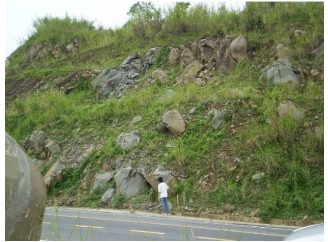
Figure 10: Circular failure (crushed) (B1 – b) at RS 10 shows the surface weakness (revealing) within the structure, which composed of coherent crushed rocks on the gently sloping discontinuities
