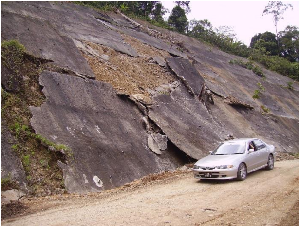
Figure 9: Complex failure (slump flow) (T5 – b) at SS 10) shows the landslide scarp above the road showing the vertical displacement
