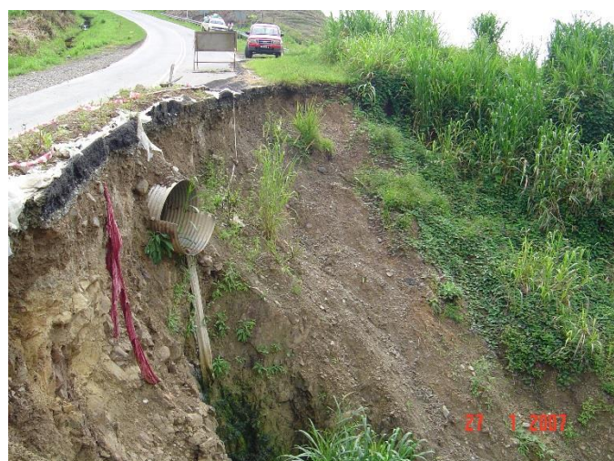
Figure 7: Embankment failure in the form of a deep slide (T1 – b) at SS 6
